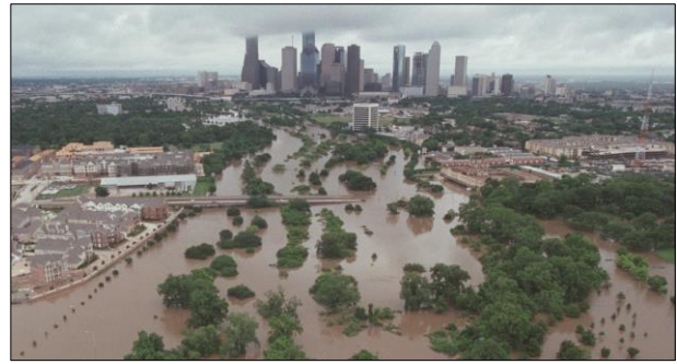
Buffalo Bayou flooding from Tropical Storm Allison.
